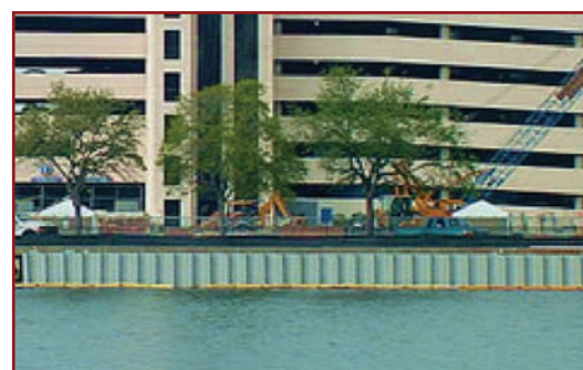
Composite Seawall, Tampa, FL
