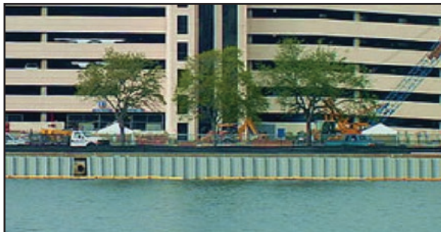
Composite Seawall, Tampa, FL
